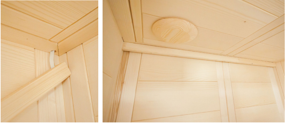
Fig. 41: Attaching the LED strip
