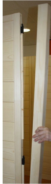
Installation of the two front corner- posts with a groove for glass
