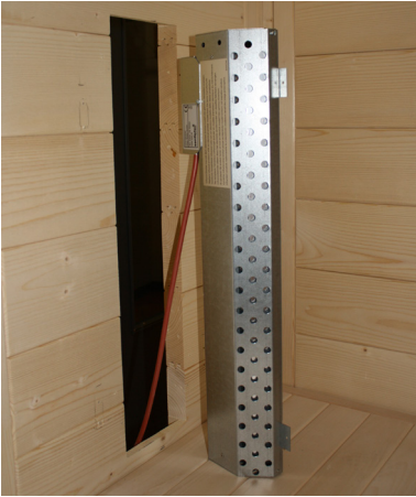
Fig. 36: Install the rear radiator (infrared radiator ECO 350)
