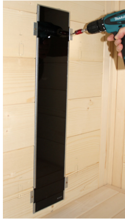
Fig. 36: Install the rear radiator (infrared radiator ECO 350)
