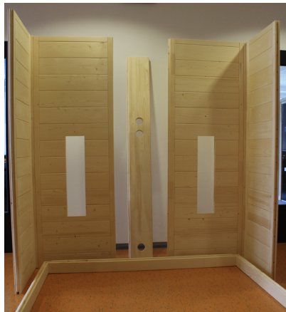
Fig. 5: Installation on the floor frame
