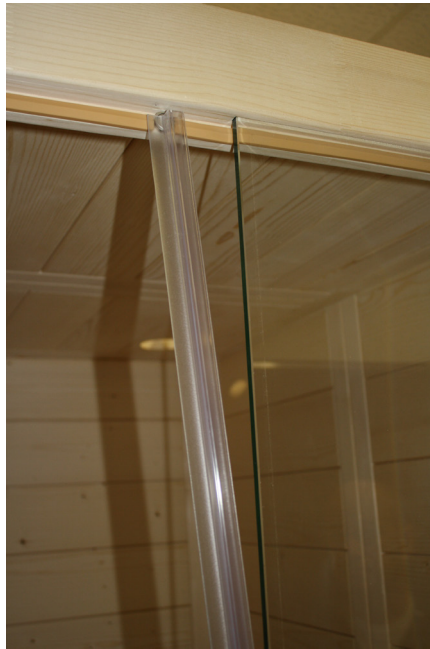
Fig. 19: Installing the door insulation strips
