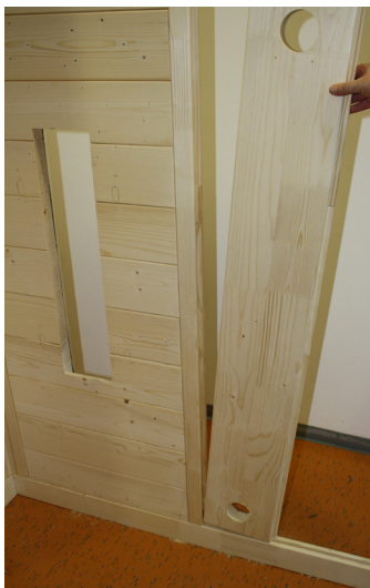
Fig. 6: Install the electrical element in place
