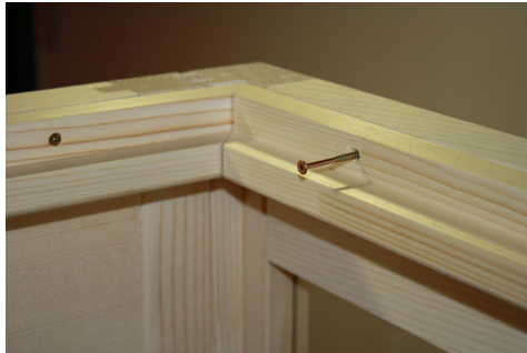
Fig. 14: Roof support slats installation
