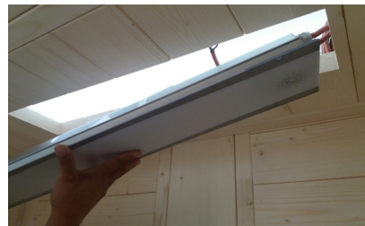
Fig. 44: Installing the colour light
