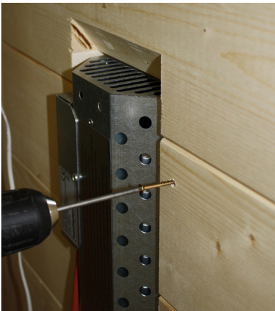
Fig. 37: Installing the read radiator blind
