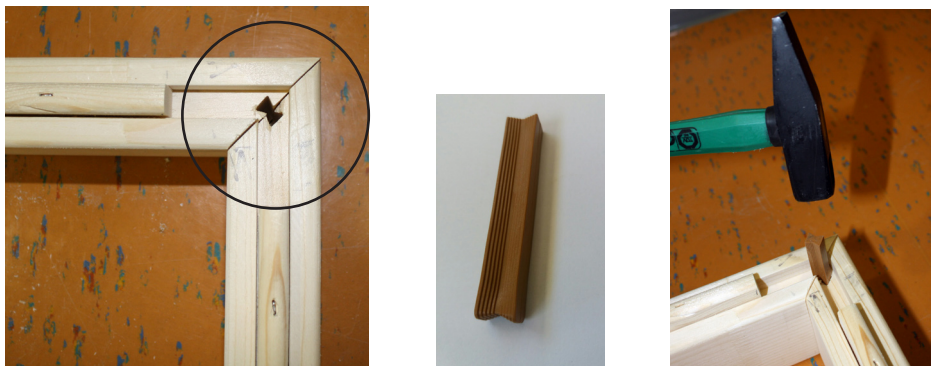
Fig. 2: Connect the floor frame elements
