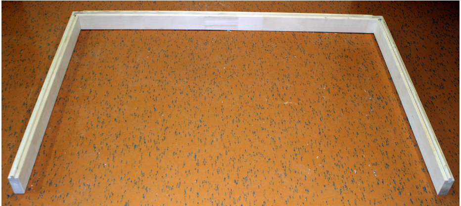
Fig. 1: Placing the three floor frame elements
