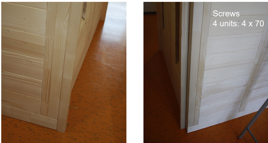
Fig. 46: Installation of the spacer strips of the rear wall
