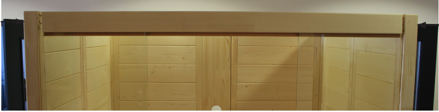
Fig. 13: Attaching the skirting
