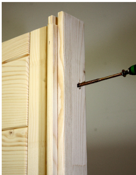
8 screws 6 x 120 mm per corner post
