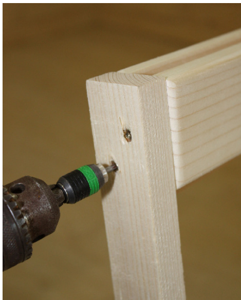
Remove transport strip from the door frame
