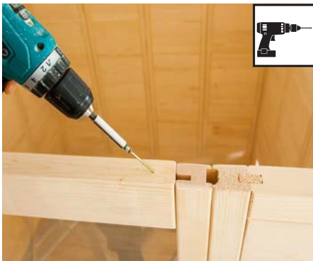
Foret de 3 mm, 1 vis 4 x 70 mm
