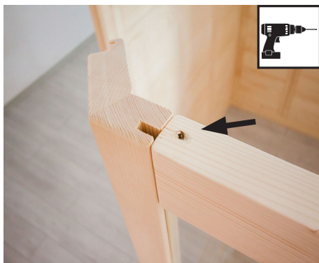
Foret de 3 mm, 1 vis 4 x 70 mm
