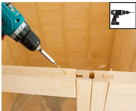
Foret de 3 mm, 1 vis 4 x 70 mm
